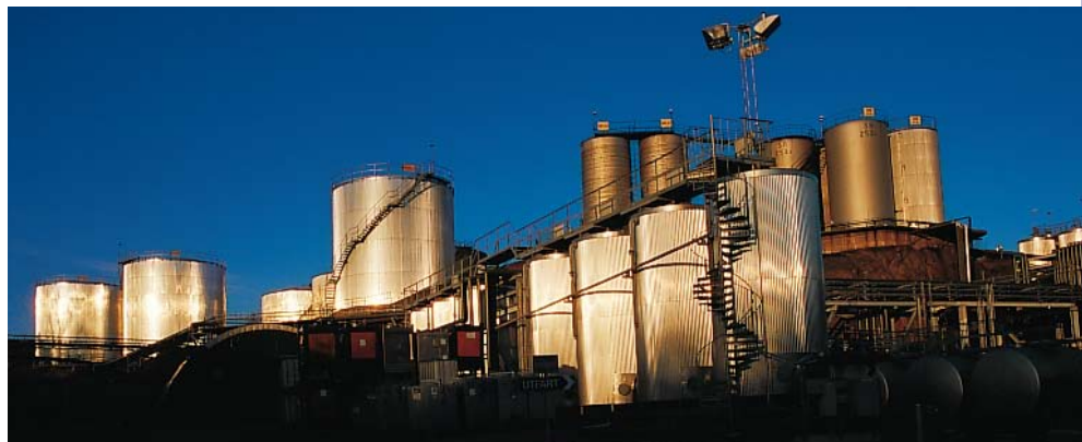
Nynäshamn — mixing plant for lubricants and main store for Sweden.
